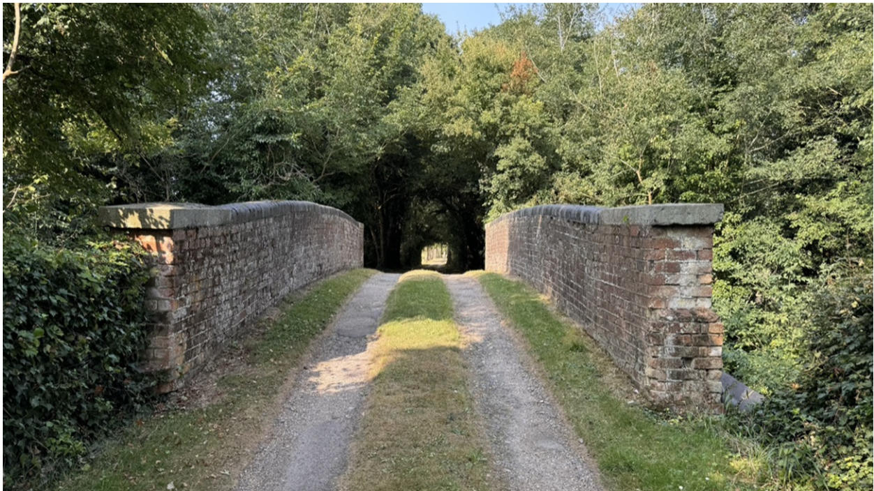
View over Bridge 2173 towards Pope Mill Farm
