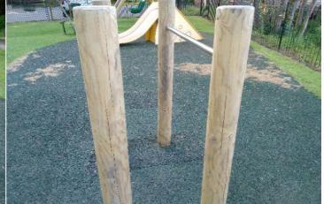
**Finding:** The timber has a number of splits/shakes or air **Action:** Monitor to ensure the splits do not cross through cracks and this may affect the stability or allow water ingress fixing points of the structure and/or cause any instability which will accelerate the rotting process
