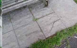
**Finding:** The paving surface under or around this unit has been damaged
